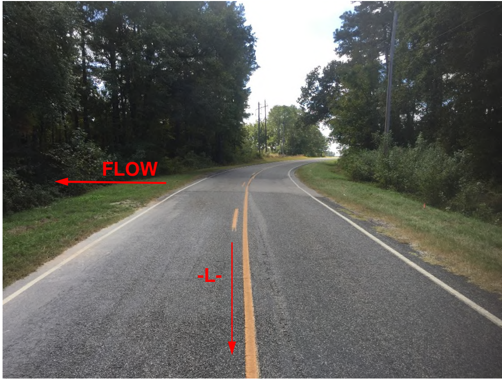
Photograph No. 1: View of -L- and Little Raft Swamp looking south.
